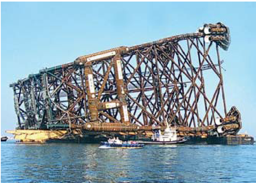
Figure 3. Typical offshore jacket structure
