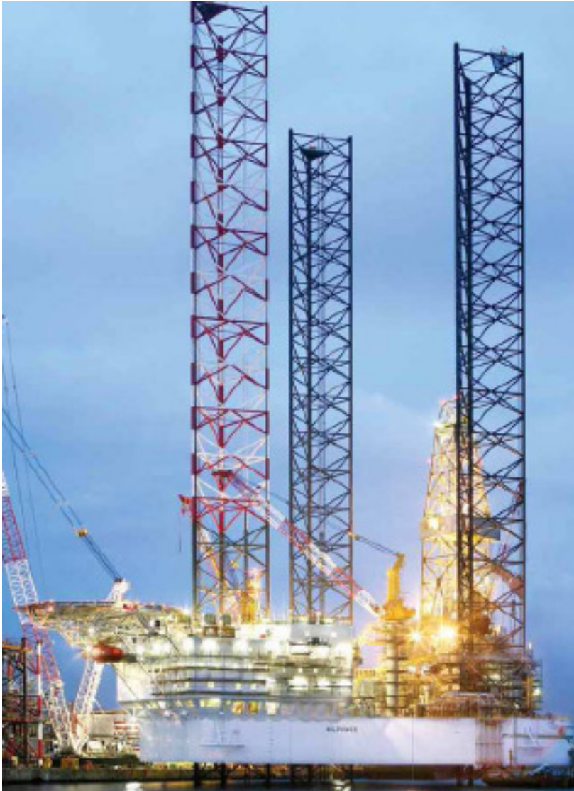
Figure 6. Jack up offshore rig.
